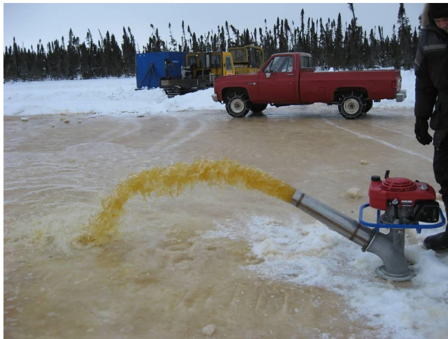
Figure 20.2: Building a thicker drill pad by flooding the ice to create lifts that freeze in 12-24 hours. © Chris Pedersen
