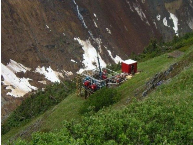
Figure 20.1: Drilling on steep slopes requires attention to drill pad stability and fall prevention. © Hy-Tech Drilling Ltd.
