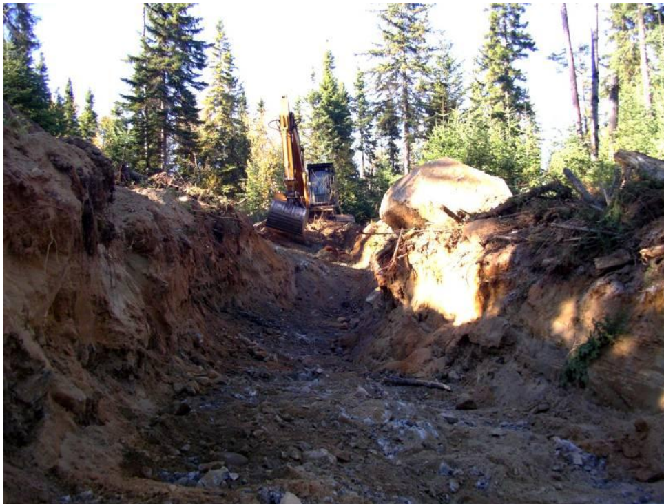
Figure 21.7: Trenches should have one end with a gentle slope for easy exit. © Lorne Burden
