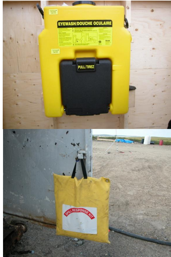
Figure 18.2 Site specific emergency response equipment: Eye wash station (left) and spill kit (right). © Bill Mitchell
