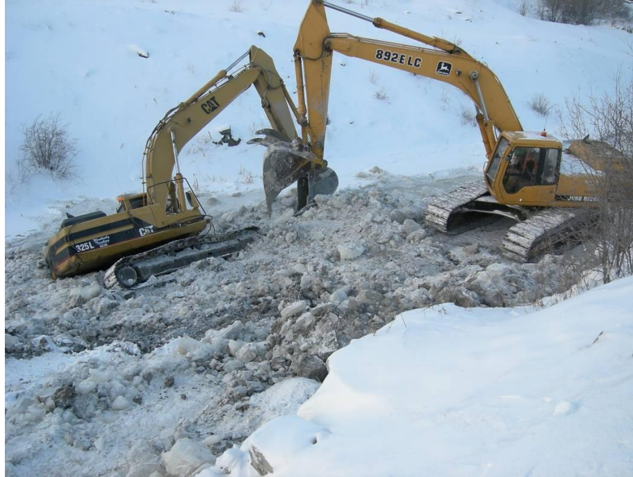
Figure 21.5: Measure the thickness before using heavy equipment on ice, especially on frozen rivers and streams where ice thickness is always variable. © Steve Millar
