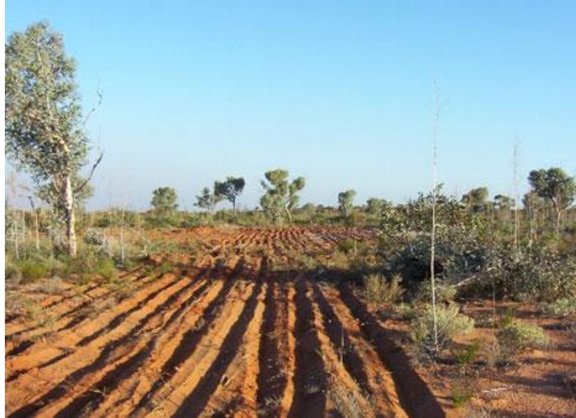
Figure 49: In parts of Australia, drill sites and access roads can be ripped or furrowed to expedite rapid regeneration of vegetation. In forested terrain elsewhere, a similar technique is called scarifying. © Mithril Resources.
