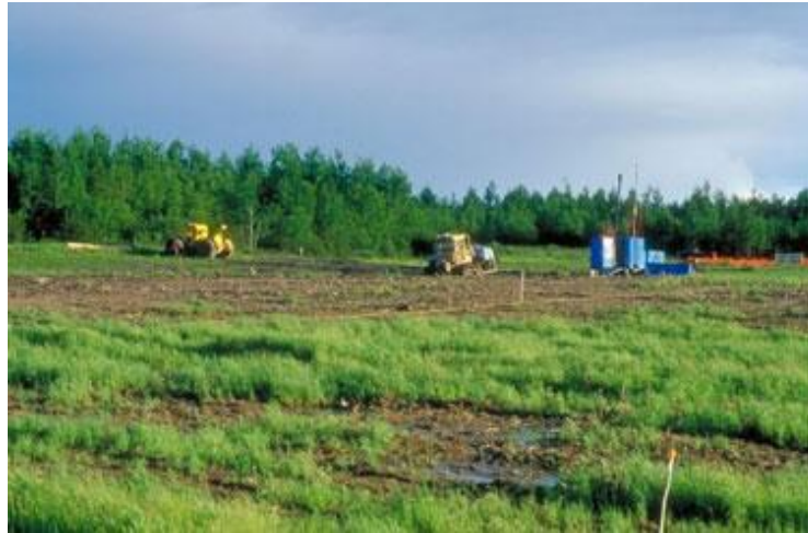
Figure28: In many regions, drill sites can be reclaimed by revegetation with local plant species after ground preparation (scarifying). © Noranda/Falconbridge
