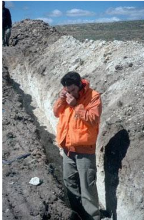
Figure 11: Trenching can leave a major scar on the landscape unless reclaimed. The muck pile from this trench in Argentina will be used as backfill upon completion of work. © Iamgold.
