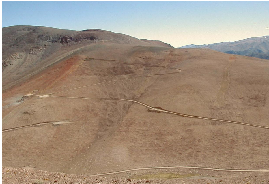
Figure 27: Drill roads and on upper left, old trench, Atacama Desert, Chile. Illustrates very slow recovery of old trenches in very arid environment. Also clear is the very visual and permanent effect of roads in this environment. (Photo courtesy Noranda 2004)
