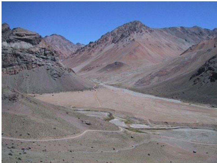
Figure 15: If well-designed, access roads can be constructed with minimal land disturbance as in this example from Argentina. © Noranda/Falconbridge
