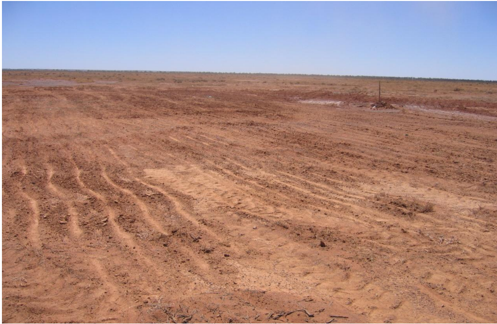
Figure 33: Reclaimed drill site using scarifying with bulldozer to encourage retention of rainwater, assist vegetation growth and reduction of erosion, Queensland, Australia, Photograph: Bill Mercer
