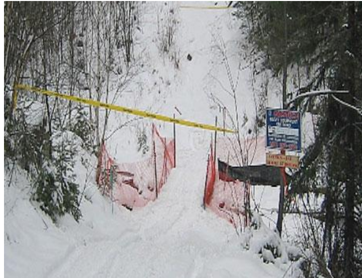
Figure 20: Winter stream crossing. Note use of snow fencing for guidance, warning signs and silt fencing. © Noranda/Falconbridge
