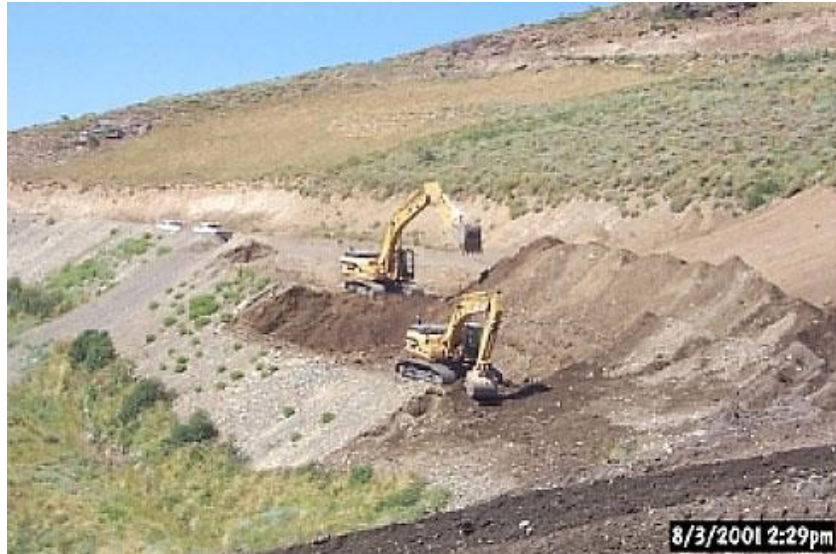
Figure 68: Road reclamation usually involves two excavators working in tandem. The original slope is restored by cutting down the upper slope and pulling up material from the lower slope. © AngloGold.
