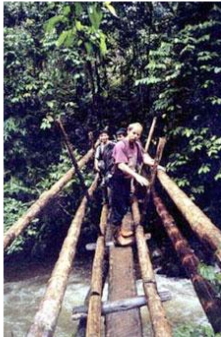
Figure 16: Bridges can be constructed from local materials and need not be major structures if equipment can be moved by hand as in this example from Central America. © Energold
