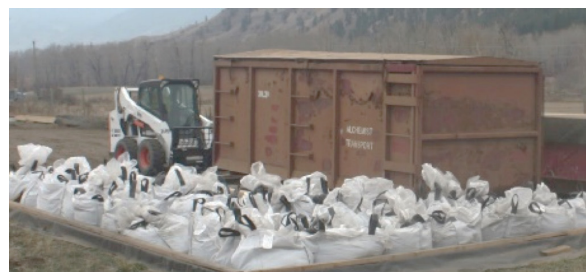
Waste from closed-loop drilling ready for transport off-site.
