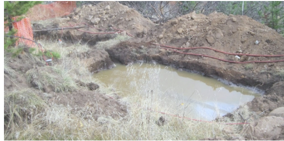
Typical sump used for waste water and drill cuttings on-site.
