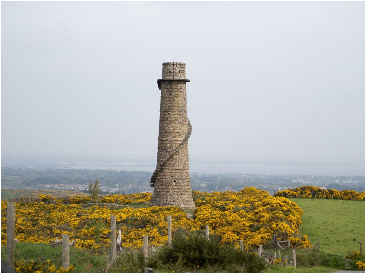
Figure 2: Exhaust chimney preserved at the historic Ballycorus Pb mine, County Dublin, Ireland.
