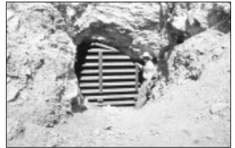
This grated adit is safe for both bats and people.
