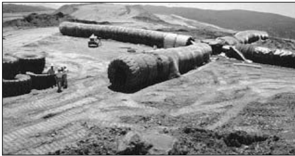
At Homestake's McLaughlin Mine, a pre-fab bat shack has been made out of 500 surplus truck tires.
